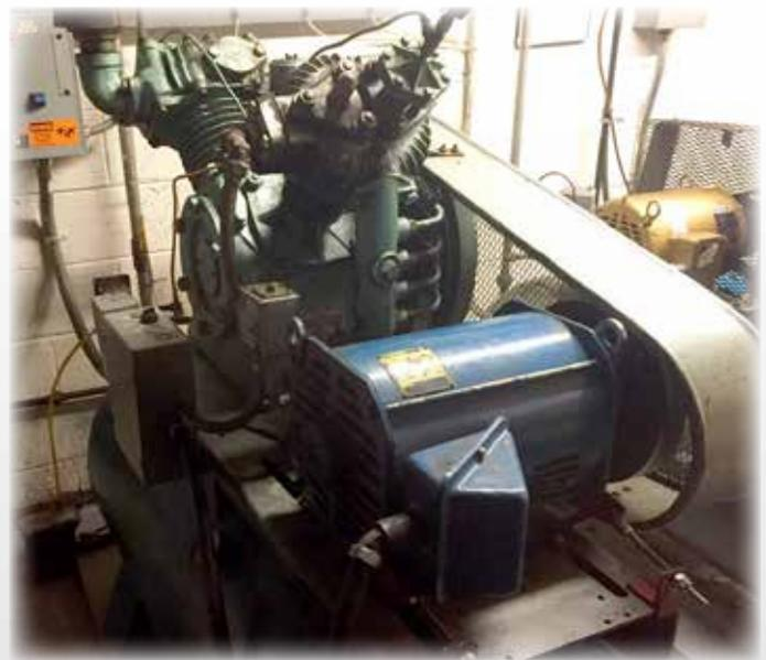
"Another benefit (provided by LE) is the LEAP<sup>SM</sup> oil analysis program. We had a high metal flag on a sample. Inspection found bearing journal wear on one shaft. We had time to procure and install a new gearbox without an hour of downtime."
